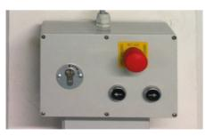
Key switch with buttons for the sliding direction and emergency-off, in dead man's control, with brief operating instructions fastened on the wall and cabling to the power unit.
