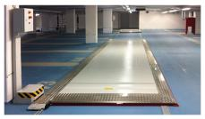
the power unit must be placed in the middle of the total platform's driving path, preferably at a column or in front of a building pillar.
