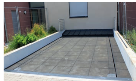
Rubber covering in stone structure (3 cm thick)
