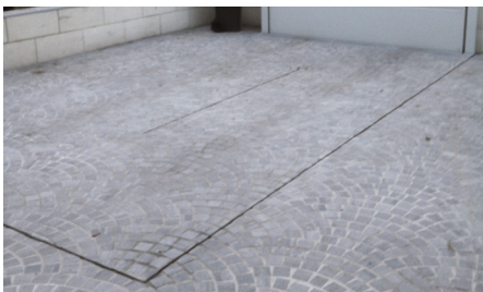
Synthetic stone covering (3 cm thick)
