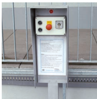
Berlin control unit with weatherproof casing and pillar
