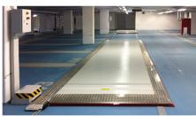
the power unit must be placed in the middle of the total platform's driving path, preferably at a column or in front of a building pillar. The switch cabinet is fastened above the power unit and cabled to it.
