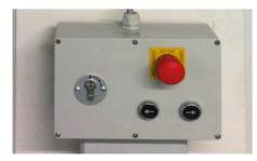
Key switch with buttons for the sliding direction and emergency-off, in dead man's control, with brief operating instructions fastened on the wall and cabling to the power unit.
