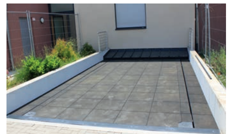
Rubber covering in stone structure (3 cm thick)
