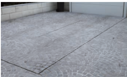
Synthetic stone covering (3 cm thick)
