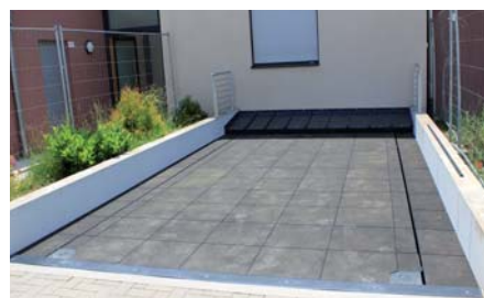
Rubber covering in stone structure (3 cm thick)
