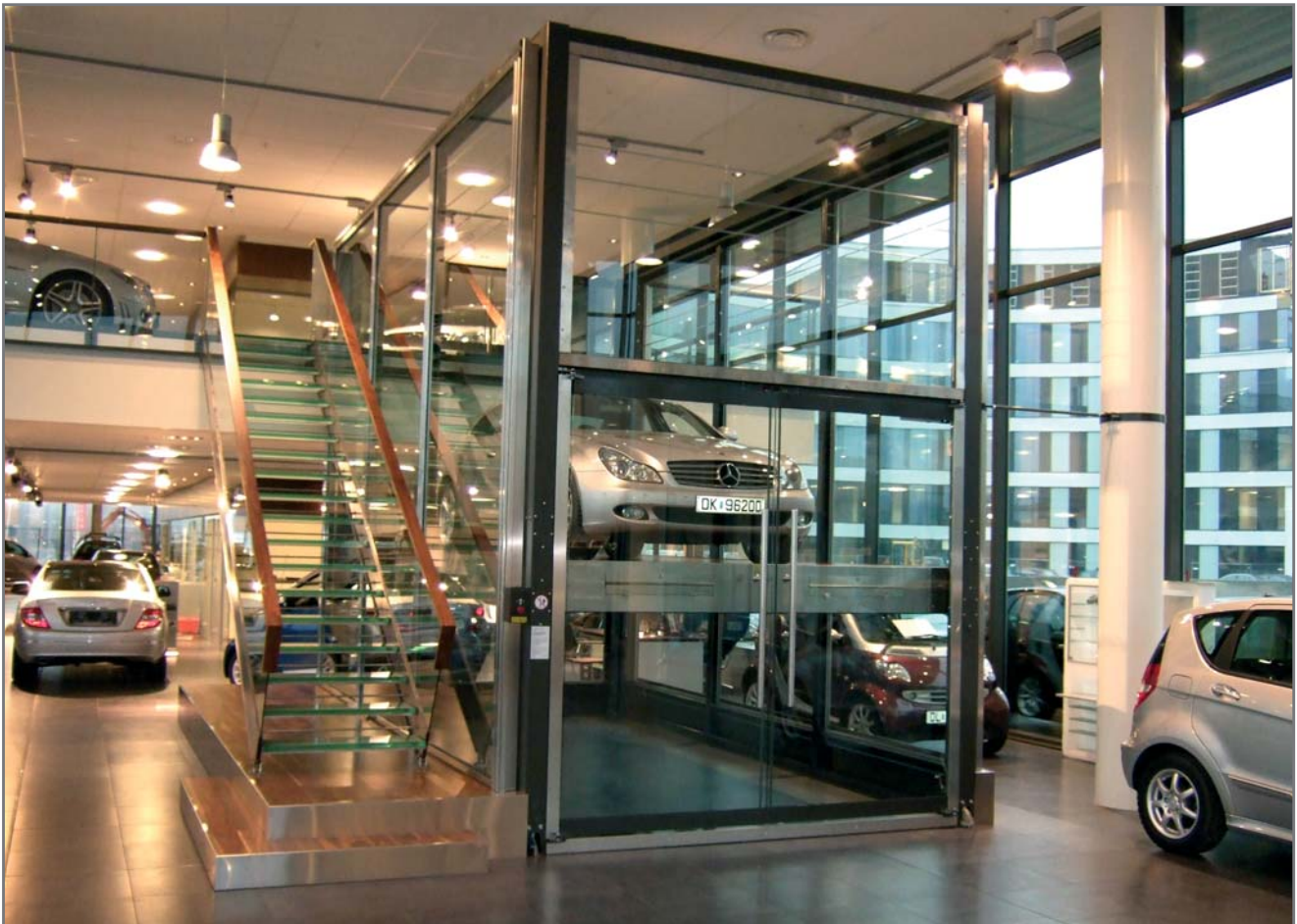
Quadro-Lift to transport vehicles to another floor
