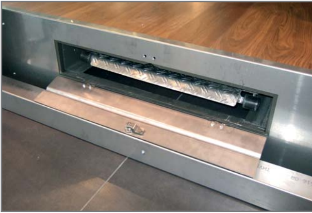
the ramp is integrated in the platform...
