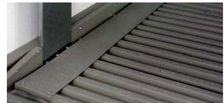
Catwalk on trapez. sheet for more walking comfort
